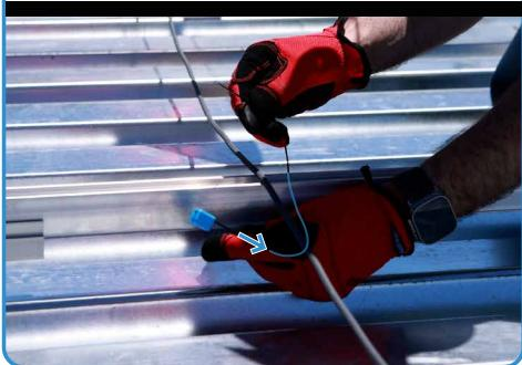
**2.** Insert into CableLoc housing.
