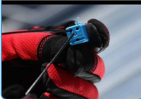
**3.** Secure excess slack with slack storage feature for future use.
